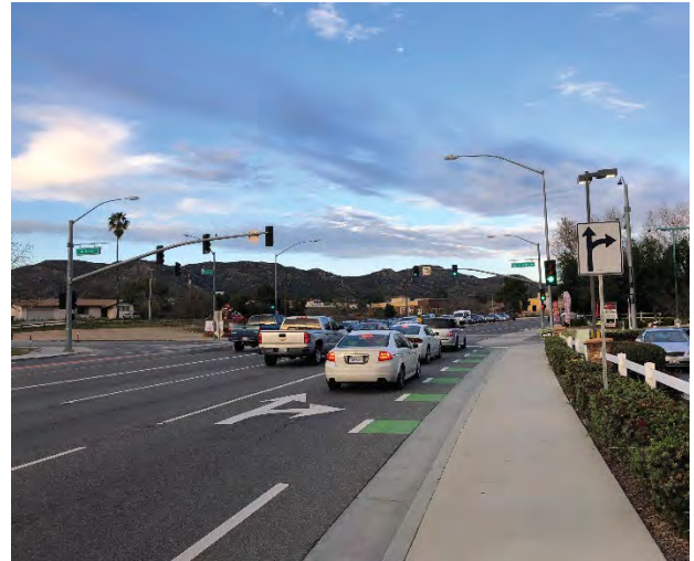
Vehicular, bicycle and pedestrian infrastructure at the intersection of Clinton Keith Road and Arya Road.
