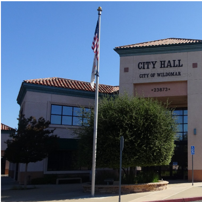
City Hall is co-located with other offices in the Oak Creek shopping center.
